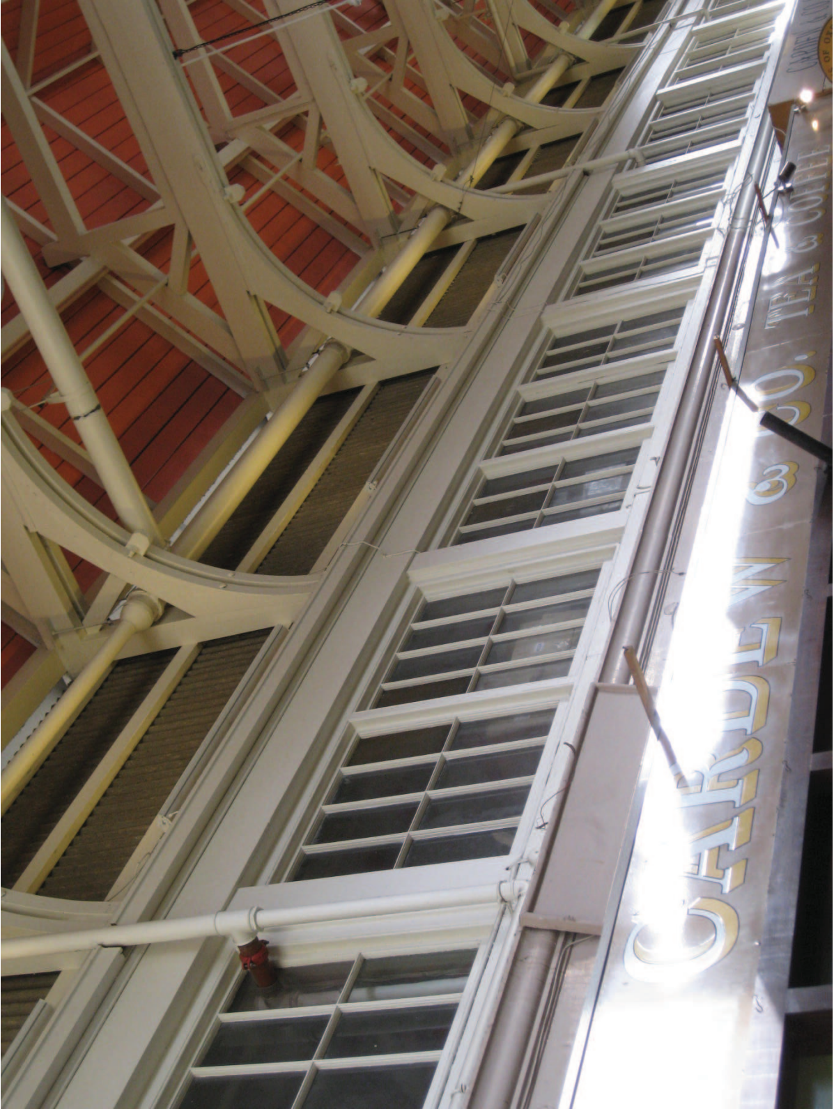
Existing: upper level glazing looking south
