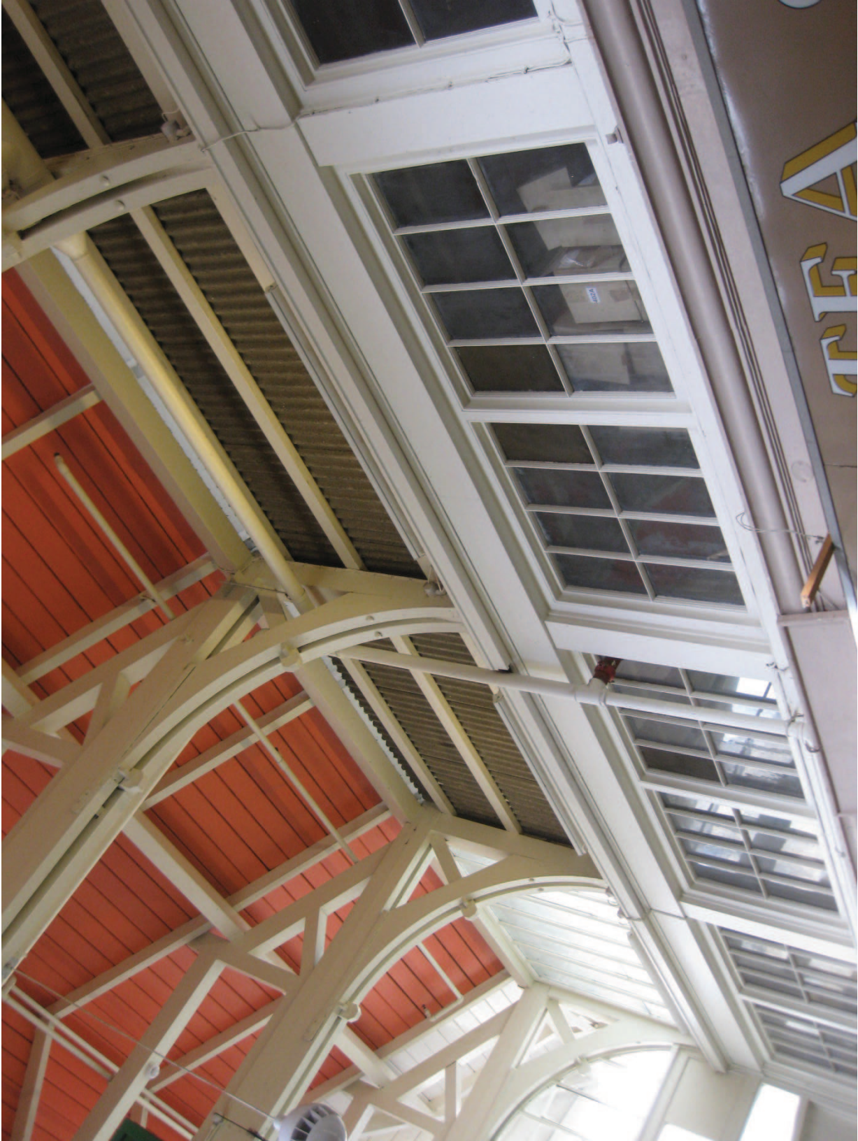
Existing upper level glazing: looking north
